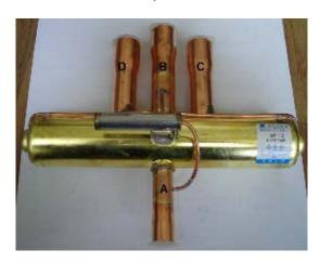
The reversing valve has four ports (A, B, C, and D):
