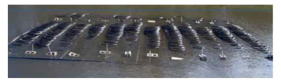
Submerged loops can be formed by coiled polyethylene pipe, mats or plate heat exchangers. Typical installations require around 300 to 500 ft. of pipe per cooling ton (27 to 45 m/kW) and approximately 3,000 ft<sup>2</sup> of surface water per cooling ton [79 m<sup>2</sup>/kW].
