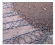
Alternative configuration to a standard straight pipe system. Coiled pipes allow access to more heat energy form a smaller area, however may require more pump energy to circulate the water/solution.
